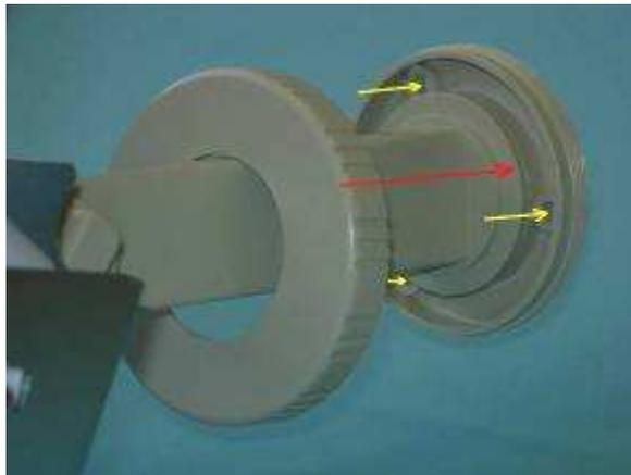
**Figure 7. Attach the mount to the wall and return cover.**
