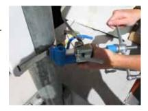
Using the built in cutting tool on the Band-It tool, cut the excess strap.
