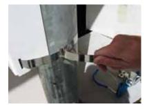
Using the Band-It tool, place the tool onto the strap.
