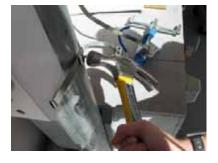
• The completed attachment should have the mounting bracket firmly seated against the pole. One band should be enough for most installations however a second band can be used for additional mounting security.
