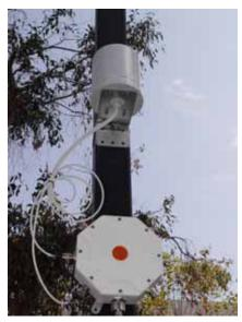
The following illustration shows a typical wall mounted XR-1000H installation after the antenna is installed and cable attachments have been completed.
