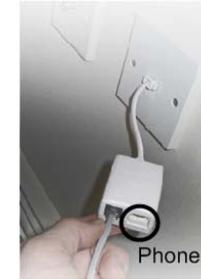
1) Plug one of the provided microfilters into your telephone socket. Any devices that were attached should then be plugged into the "Phone" socket of the microfilter.
